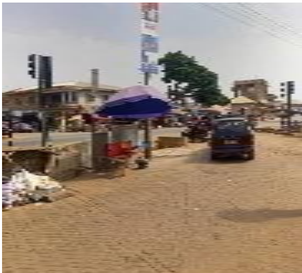
Construction and installation of 1No.traffic light facilities at Duayaw Nkwanta
