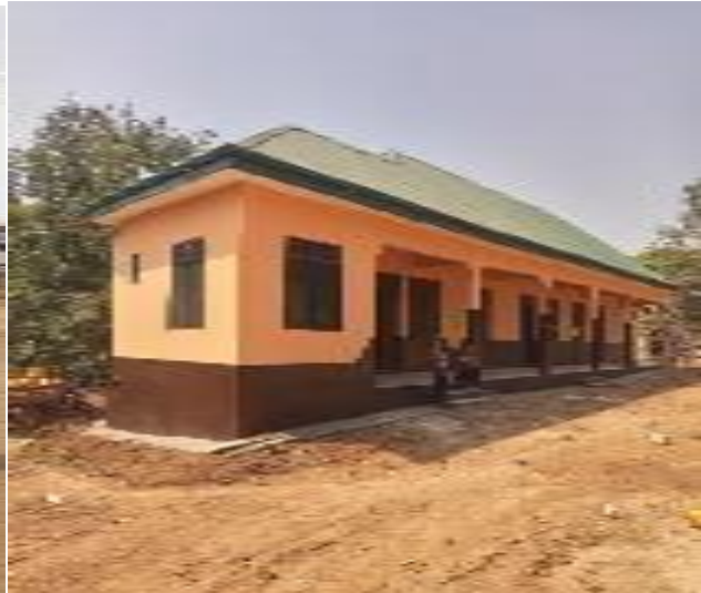
Construct 2 unit KG block with ancillary at Twabidi
