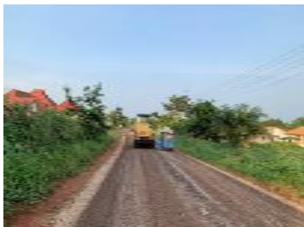
Complete the Bitumen surfacing of residency road Duayaw Nkwata
