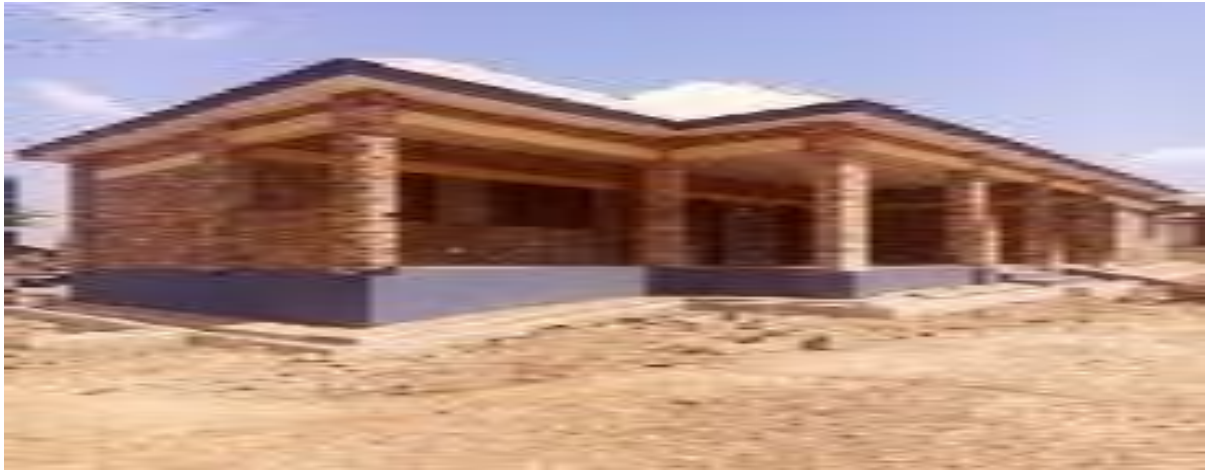
Construction of 1No. Maternity Block at Mankraho
